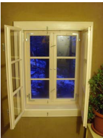
Figure 1-c. Double glazing with large spacing (from fachwerk.de)
