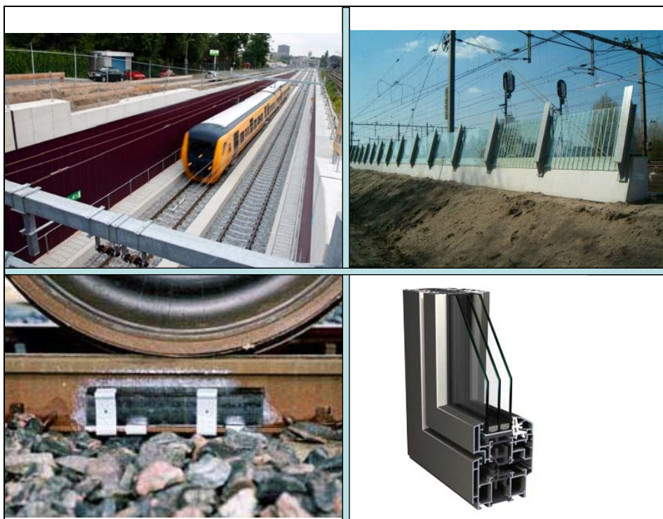
Figure 1-b. Options for noise control by the infra manager. Clockwise from top left: alignment (cuttings and tunnels), barriers, façade insulation, track measures (rail absorbers)
