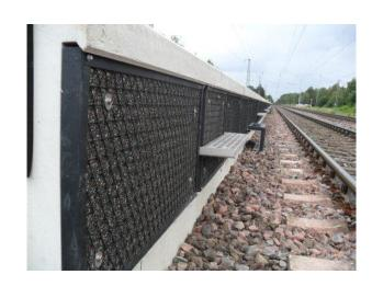
Figure 15 (left): Zbloc barrier.
